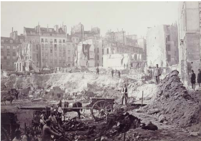
Charles Marville (known as Charles Bossu), Construction of Avenue de l'Opéra. Worksite on Rue d'Argenteuil, near Rue du Faubourg-Saint-Honoré, December 1876
