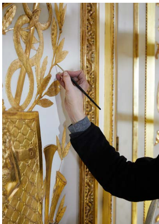
Drawing Room of the Hôtel d'Uzès undergoing restoration © Antoine Mercusot
